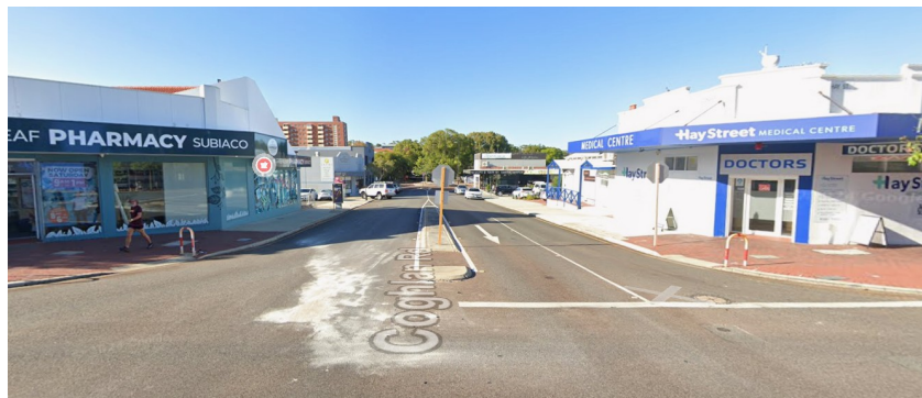
Coghlan Street looking south
