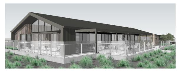
The building itself includes a mixture of feature timber cladding, stone wall cladding and metal/aluminium paint finishes in 'Woodland Grey'. Extensive glazing is incorporated to enhance natural light into the building and ensure visual permeability to the surrounding public realm.
